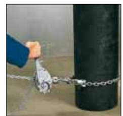
Hoist with sling chain
